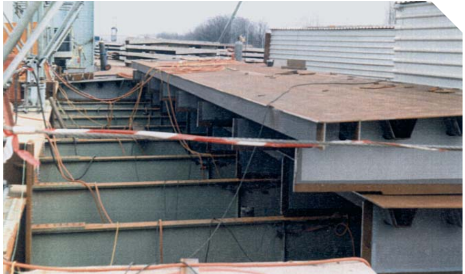
► The Rodenkirchten bridge, showing the confined spaces under the main decking.
